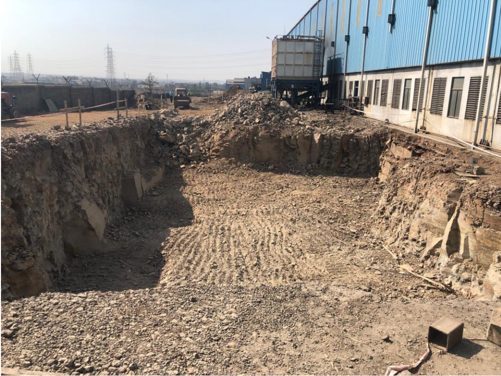
Furnace & Raw Material Storage Pit Foundations
