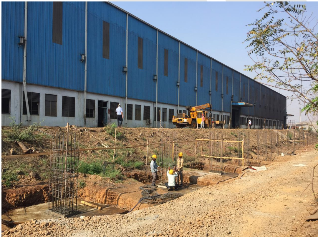
Building Foundation in Progress
